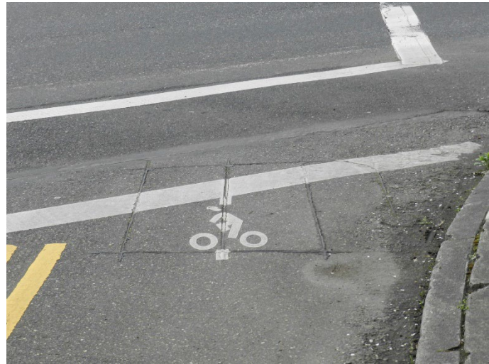
A bike detection loop and marking to indicate where a bicyclist should wait.
