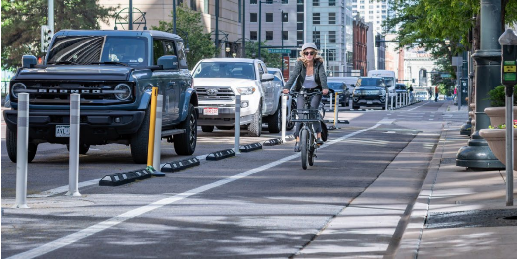
Intermittent vertical elements (flex posts and curb stops) along a separated bike lane
