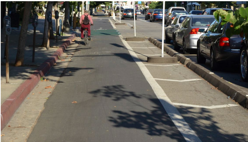
Continuous vertical elements (concrete curb) along a separated bike lane
